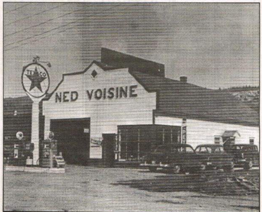
Market Street Motors was located at the current site of Herman and Claire Theriault's C.N.A. Trucking and Theriault Boys, Inc. garage on Market Street in Fort Kent. The service station and used car dealership was owned by Ned Voisine of Fort Kent until the time of his death at the age of 35 in 1956.
