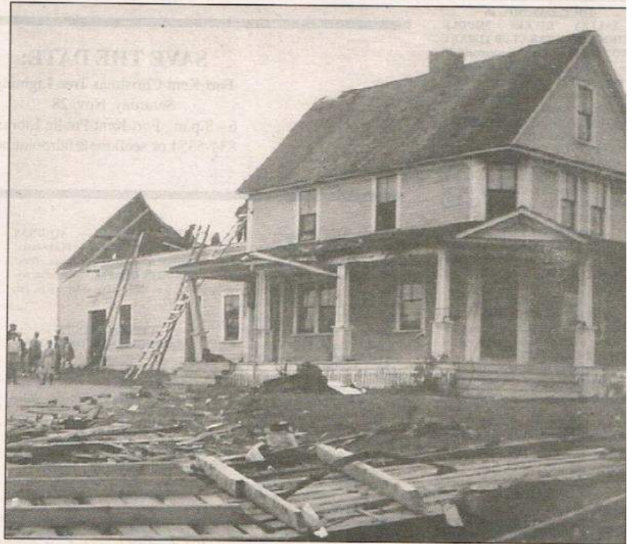
A crop duster plane came into contact with Arthur Cyr's house in the late 1930s, causing a portion of the roof to tear off.
