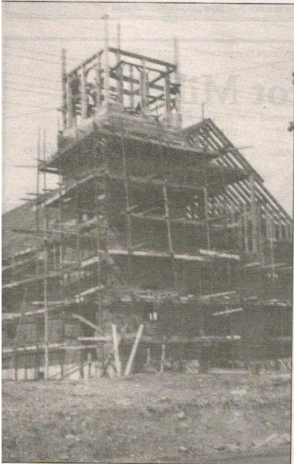
Construction on St. Gerard Church began in 1931.
