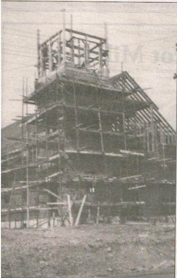
Construction on St. Gerard Church began in 1931.
