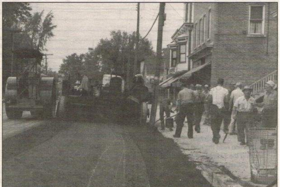
A paving crew lays down the first layer of asphalt on Main Street in Van Buren in 1953.
