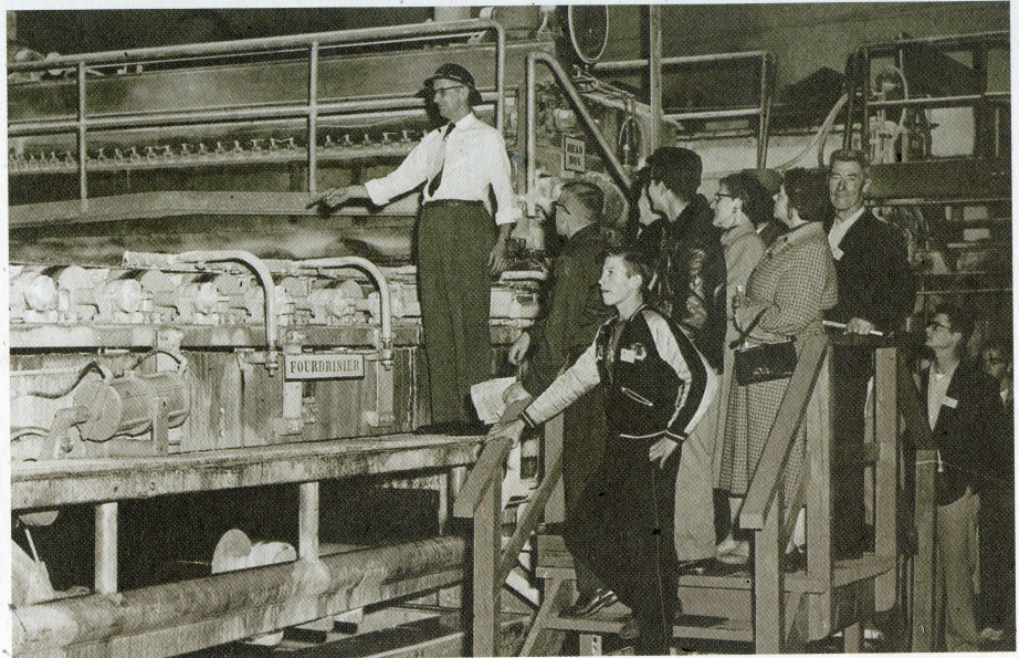
1955 - Open House guests look at Bond Mill Fourdrinier which filters water out of stock before going to the presses.
